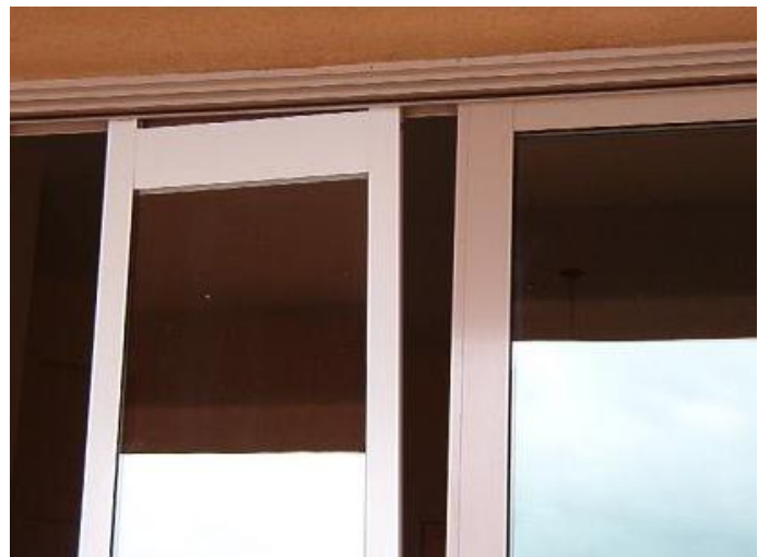
Test fit the panel insert into place.
