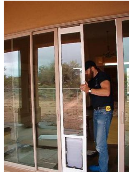
Push panel unit tight against the door jamb lip to screw into place.
