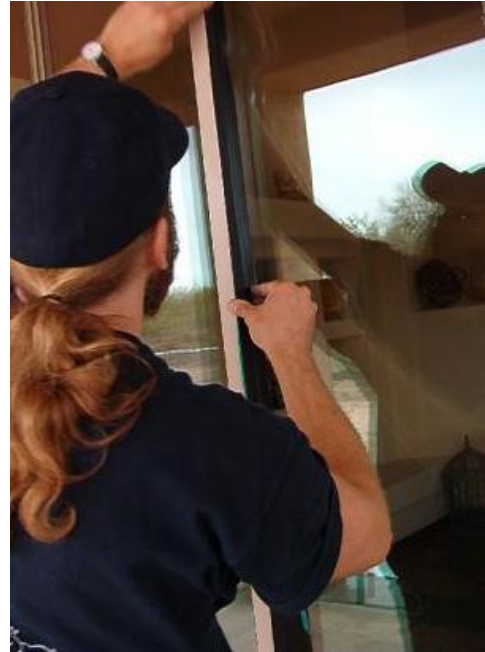
Apply vinyl weather-stripping.
