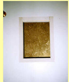
Frame the inside and outside of the hole on the door - use 1/4" cedar or pine 2" wide.
